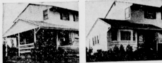
BEFORE: Carport, with roof above and slab below, was the logical spot to add living space to this three-bedroom house overflowing with family of seven. AFTER: new addition does double duty as family room and bedroom for teenager.
