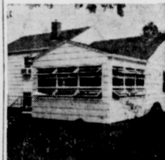
AFTER: Owner added porch by breaking through dining room window. Stock awning windows of ponderosa pine provide maximum ventilation.
