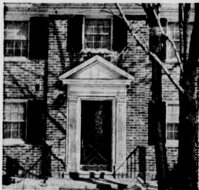
Residents of garden apartments like this one are able to live in distinctive settings because factory-made building components have made it easy for builders to add variety to apartment designs. Stock panel door, entrance, windows and shutters of ponderosa pine are used here to establish a Colonial atmosphere.
