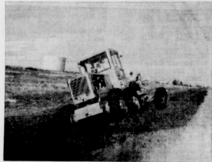
A BAR DITCH BEING DUG AT AN INDUSTRIAL SITE . . .
