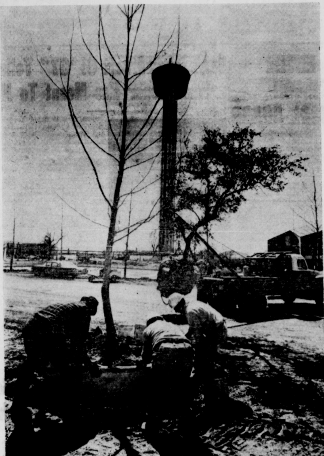
LANDSCAPING GOING IN—HemisFair workmen are planting trees and grass in preparation for the opening of the world's fair April 6. Workers above are putting the final touches on one tree planting while a truck stands ready to lower another in the continual preparation for the six-month international exposition.
