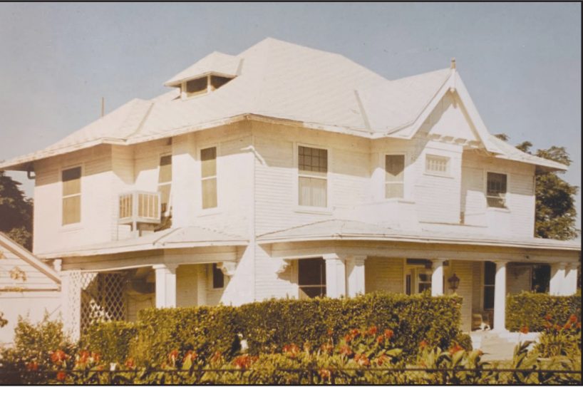
Courtesy Photo Pictured above is the Price's home at 800 Main that burned down four years ago due to an electric fire.
