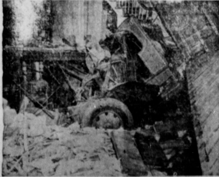
The driver of this truck lost control of it because its brakes were defective. It ran up on the sidewalk and plowed through the side of a house, killing two persons. In addition to the terrible toll of motor vehicle deaths and injuries last year—33,500 killed, 1,150,000 injured—the total economic waste amounted to almost two billion dollars. Brakes, tires, lights, windshield wipers, and other safety features should be periodically checked as a safeguard against accidents. A recent nationwide testing program disclosed mechanical defects in one out of every three cars examined.
