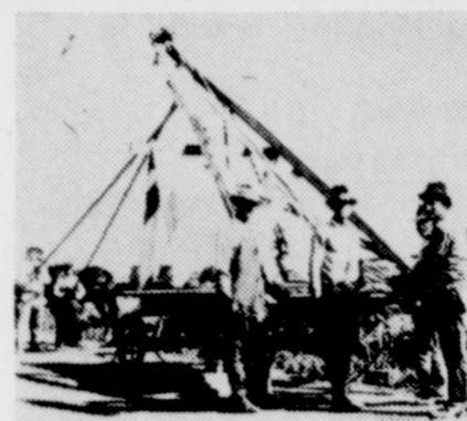
50 years ago, the year Southwestern Public Service Company was born, raising transmission poles was, literally, a matter of horse and man power as pictured above. In the company's golden anniversary year, it's just a question of lift, set and tamp, as seen at right, nearly all of it done mechanically.
