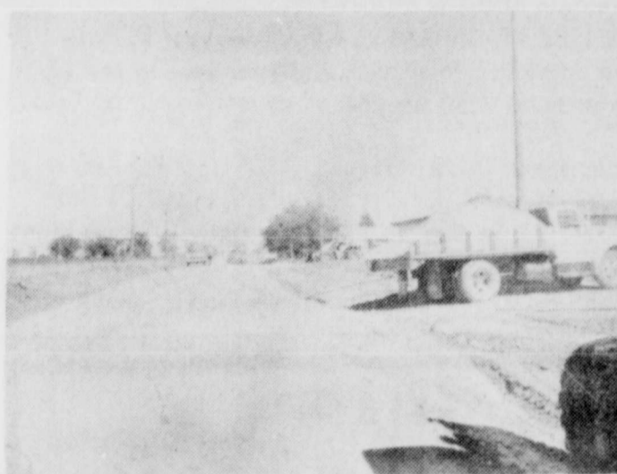
"Work in Progress on West Road" West-Side Road Improvement
