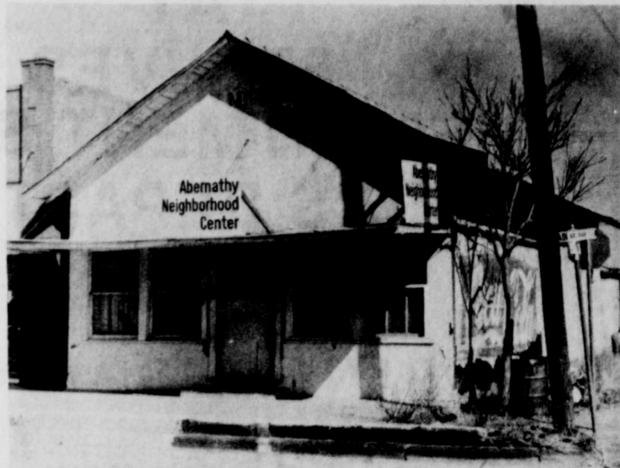
THE ABERNATHY NEIGHBORHOOD CENTER was forced to close recently due to having no more money to finance it. Pictured is the building used as the Center for the past 12 years. (Review Photo)
