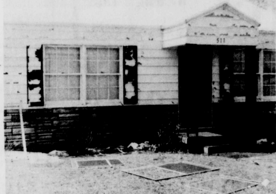
THE NORTH FACE of many houses in Abernathy received heavy damage, such as the house pictured in which the paint and outer surface were removed as well as the windows and panes broken. (Review Photo by Manny Martinez)
