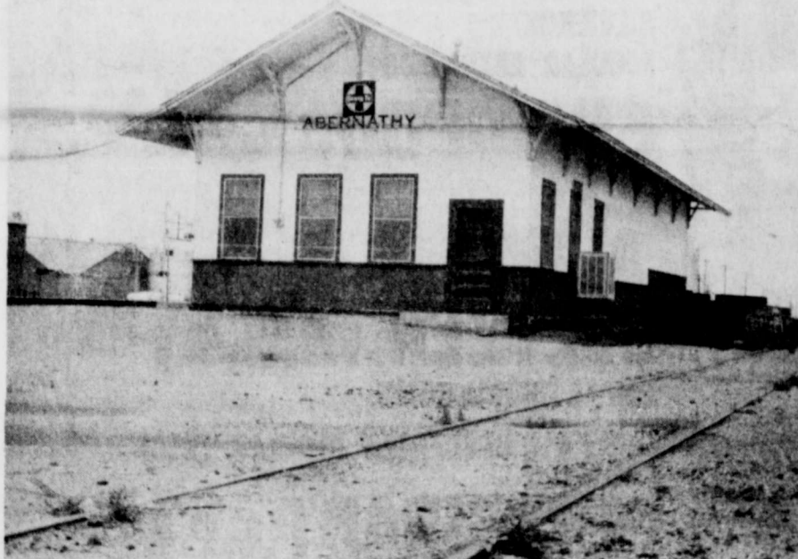
THE ABERNATHY CHAMBER OF COMMERCE has high hopes that Santa Fe Railroad Company will grant the local depot to Abernathy. Under Santa Fe policy, the structure has to remain where it is for a period of one year after it has been closed. When a year has passed, the depot will either be removed by Santa Fe or given to Abernathy. (REVIEW PHOTO)
