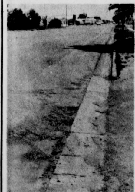
POT HOLES CAN STILL BE SEEN on Avenue D, which were caused by the heavy snow storms this winter. The Highway Department is responsible for maintaining Avenue D. (Review Photo)
