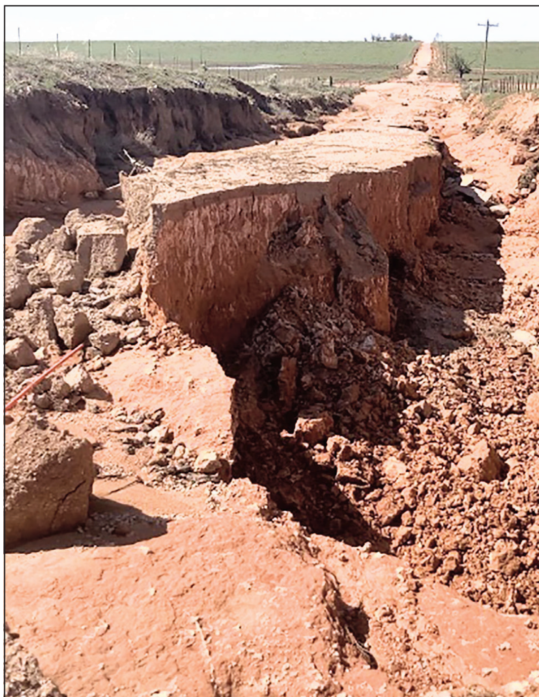
Commissioner Charles Wilkins took this photo of a washed-out county road near Bovina.
