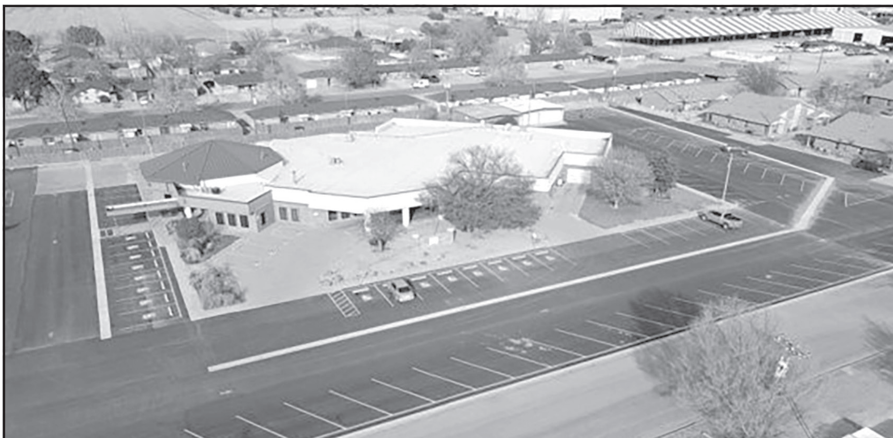
Drone's Eye View —The expansive parking lot project at the Hereford Senior Citizens Center is shown in this drone photo. Reworking of the once-potholed area around the structure is now complete. (Drone photo courtesy of Blaze Bermea)
