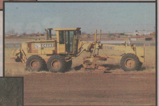
Road Building & Material Hauling
