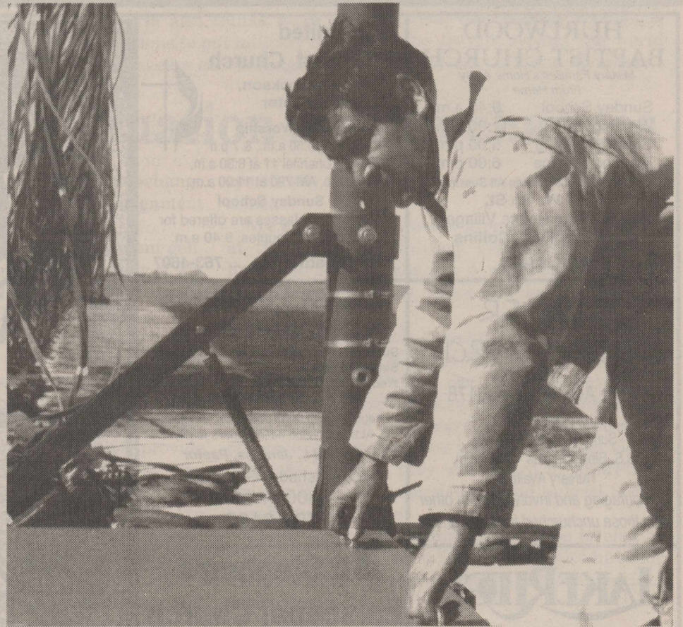
Adam Huerta, 64th Civil Engineer Squadron, makes one of the daily maintenance inspections on the BAK-15 barrier system. Above, a view of the erect barrier at the end of the Reese runway. Below, an artist's drawing shows how the BAK-15 barrier slows and stops jet aircraft.
