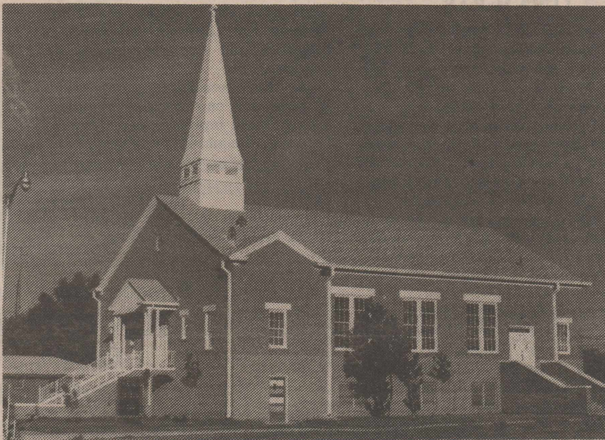
Silverton First United Methodist Church 1891-1991
