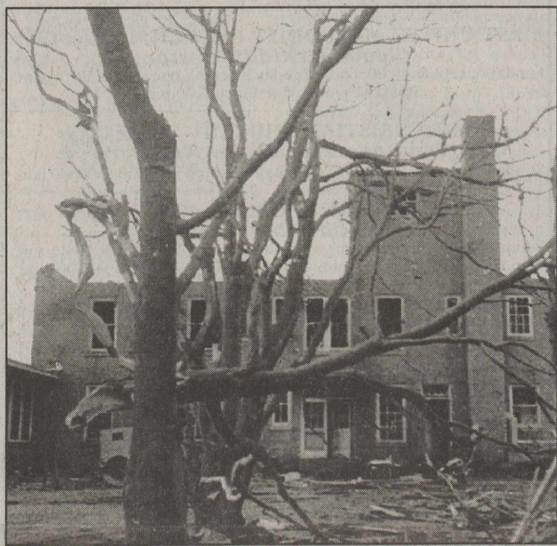
The Knox County Hospital building following the tornado that struck Knox City on Friday, March 13, 1953. The building was just one of many struck by the tornado. Thirty five blocks of Knox City felt the wrath of the storm. (Bill Baker photo)
