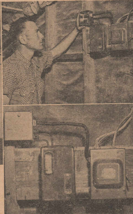
LeRoy Hutton raised 2,000 baby chicks under heat lamps with an automatic alarm unit. An overloaded circuit in the brooder house caused a fuse to blow, thereby interrupting the flow of electricity and causing Mr. Hutton's alarm to sound off about 3:00 a.m. the first night that his heat lamps were connected. Now Hutton rests well at night, knowing that his alarm will warn him of trouble in the brooder house.
