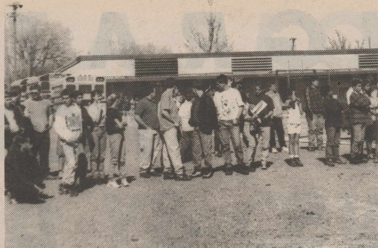
Students watched with interest as the old field house was demolished last Thursday. They are registering their guesses as to how many truckloads will be required to remove the rubble from the scene.
