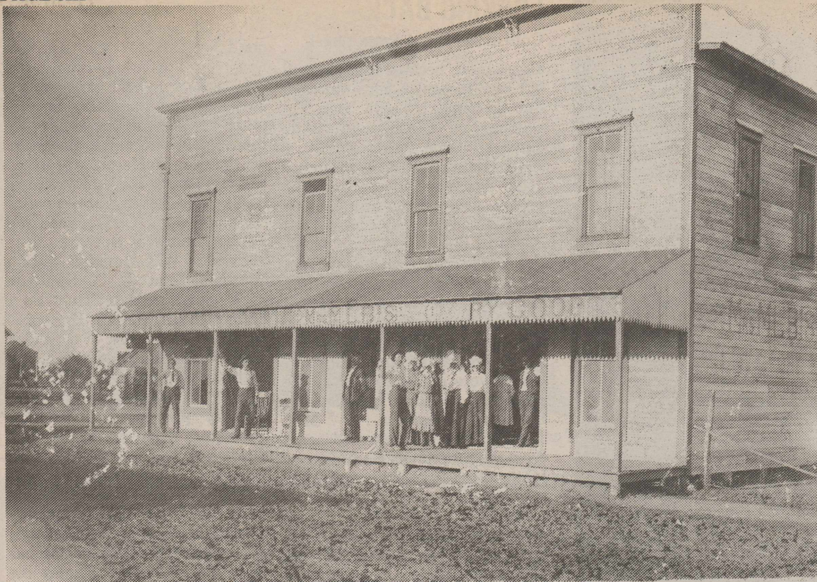
Old Lodge Building and Post Office in Silverton.
