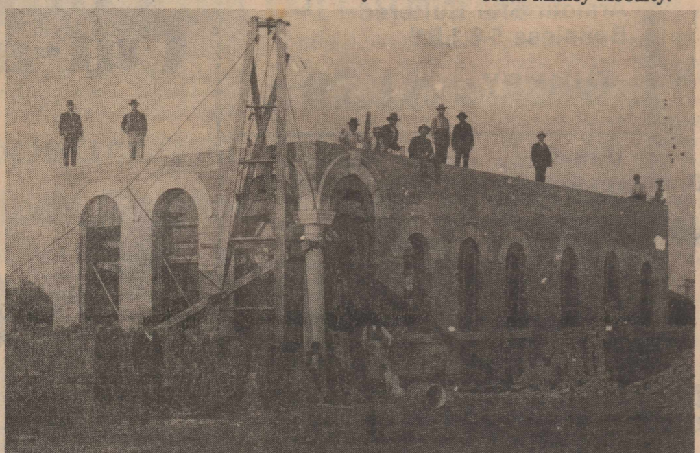
BANK CONSTRUCTION: The above photograph shows the Sylvester Bank being constructed back in the early 1920's.
