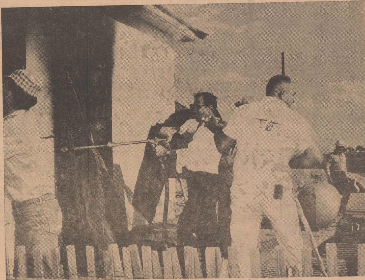
In the panel above firemen are shown braving intense heat to battle the blaze which razed the Short Whitley home in south Olton a week ago Thursday. The butane tank in the background was subsequently removed as a preventive measure. Firemen were hampered by lack of water. In the panel at left the home is a sheet of smoke and flame. It was burned to the ground. Only a few of the family belongings were saved.
