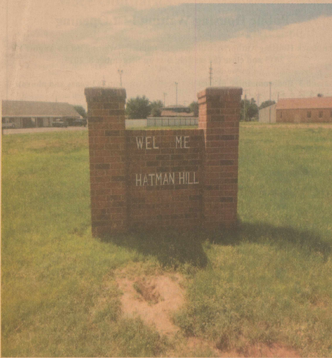
SURELY, THERE ARE THOSE WHO WANT TO SEE THIS CORRECTED! This photo was published in the August 6, 2015 edition of the Southwest Digest, and comments were received about getting it corrected. This sign is located at the corner of Birch Avenue and East 19th Street.
