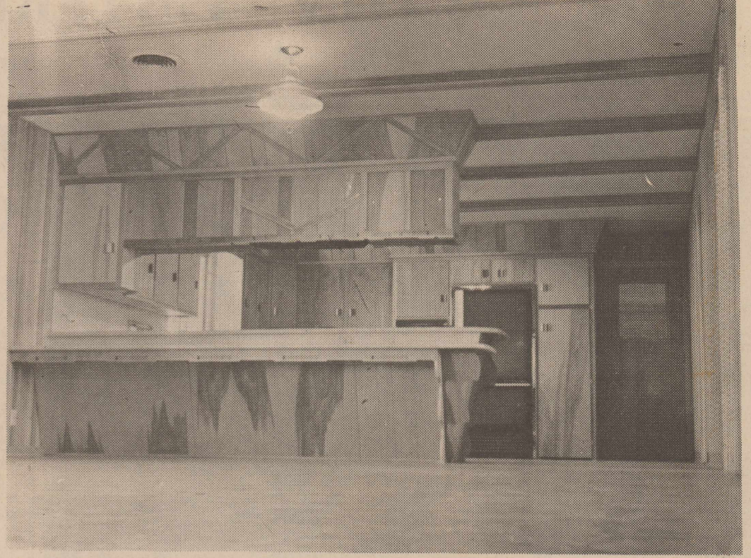
OPEN BEAM CEILING and Parana Pine and Birch paneling highlight the kitchen-den combination at the new Medallion home. A rock pattern Armstrong vinyl was used for floor covering.
