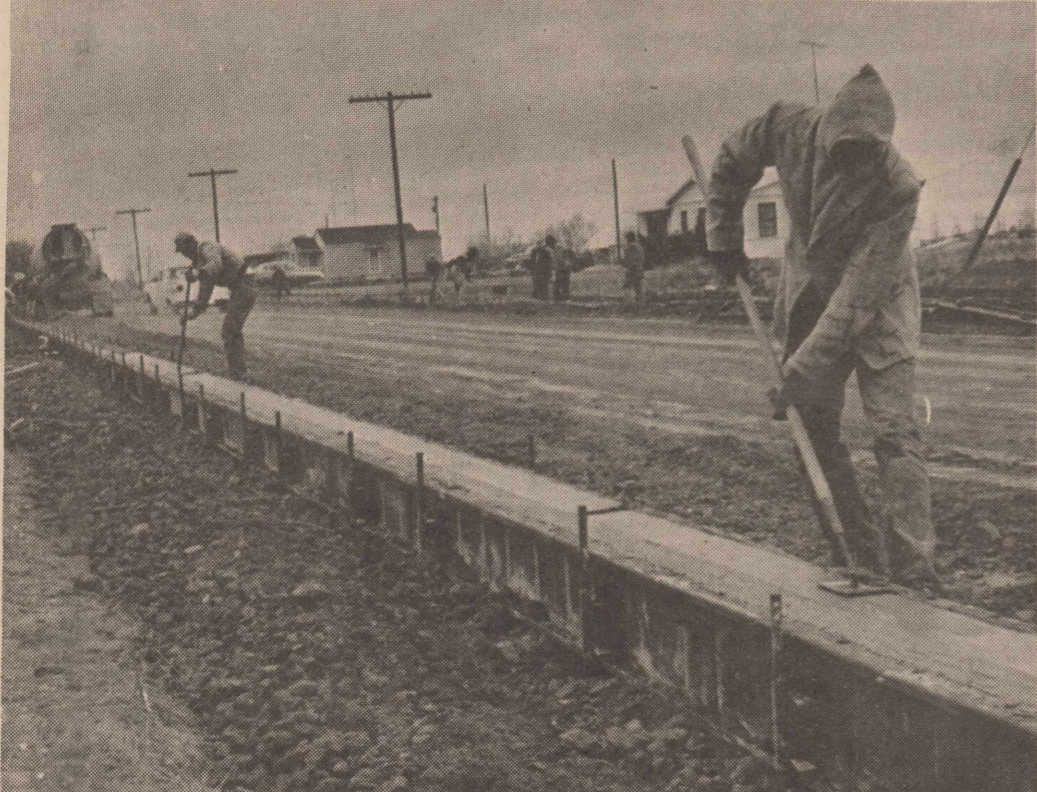
CURB AND GUTTER WORK on Olton's paving project began this week starting on West 7th Street. Shown here are workmen of Hodges and Tierney Co., Lubbock contractors, as they smooth up just-poured concrete. Forty blocks have been approved for paving by the city council, with more expected to be added as the project continues.
