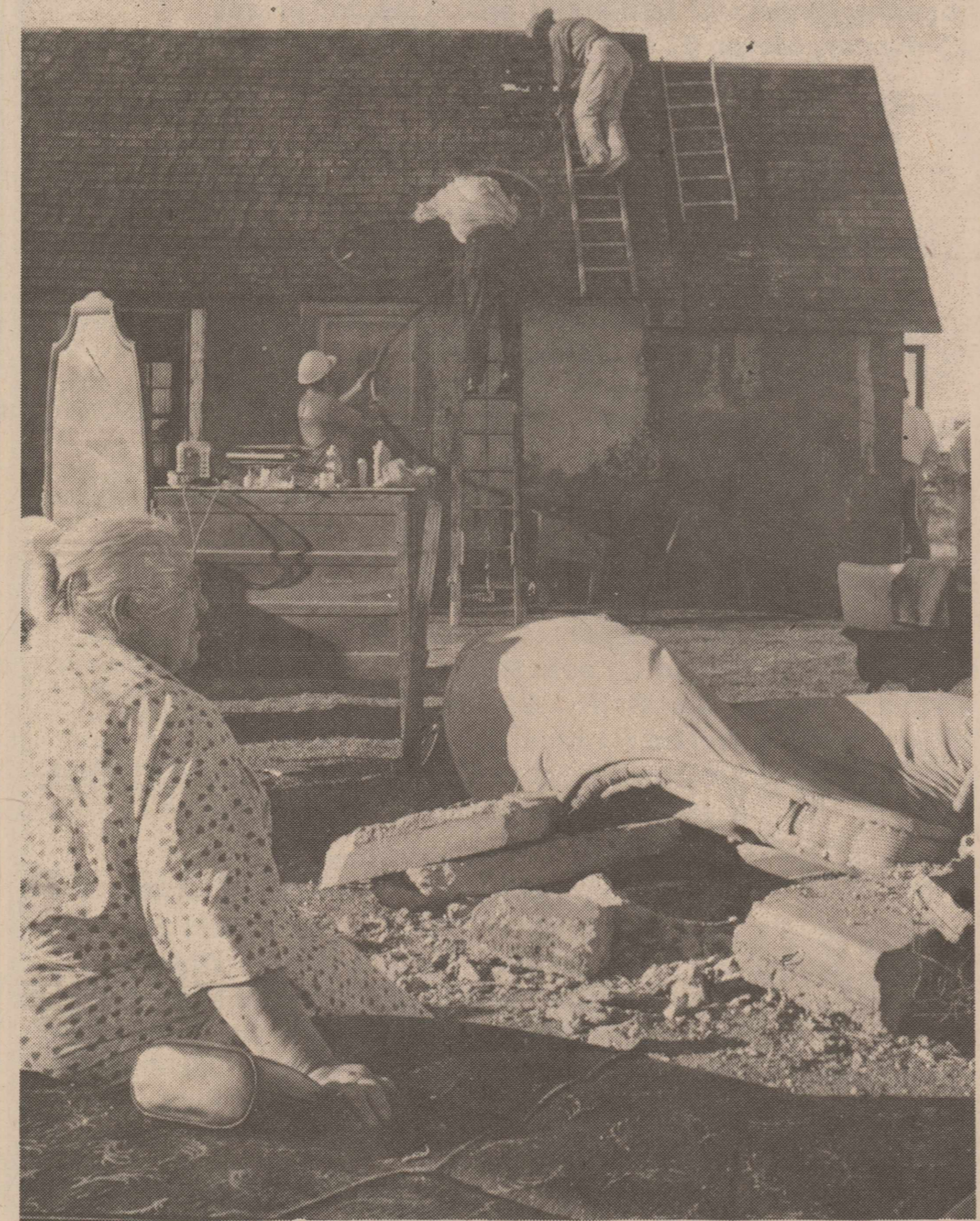
TOO HOT IN THE HOUSE ---Mrs. Charley Meyer sits dejectedly on a couch outside her home here Monday afternoon as firemen finish putting out a blaze which damaged the roof and attic of the house. Furniture was moved outside by firemen, saving it from smoke and water damage. Faulty wiring was blamed as cause of the fire. The blaze was one of three battled by firemen here Monday and Tuesday.
