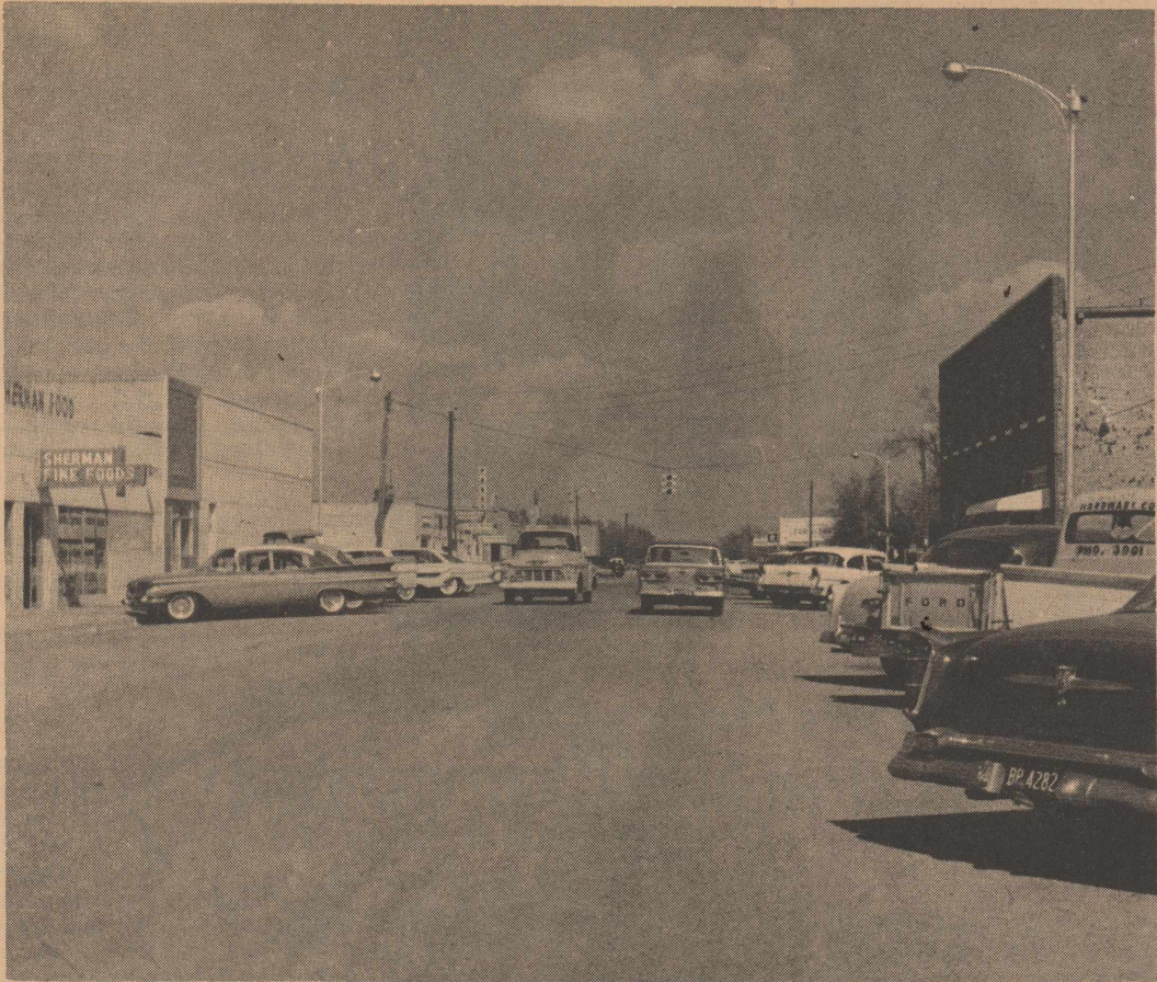
SCENE OF PARKING QUESTION---This street, 8th between Main and Avenue G, is the one on which city councilmen recently laid plans for parallel parking, vs. angle parking as shown. The street, 60 feet in width, now allows clearance as shown in the picture. Some members of the city council believe it should have more, for safety reasons. Some downtown merchants, however, are asking that the street be left as it is, saying they feel there are no undue safety hazards at present and pointing out that very few accidents have occurred there. A petition asking that the matter be given further study is being circulated and probably will be presented at the next council meeting.
