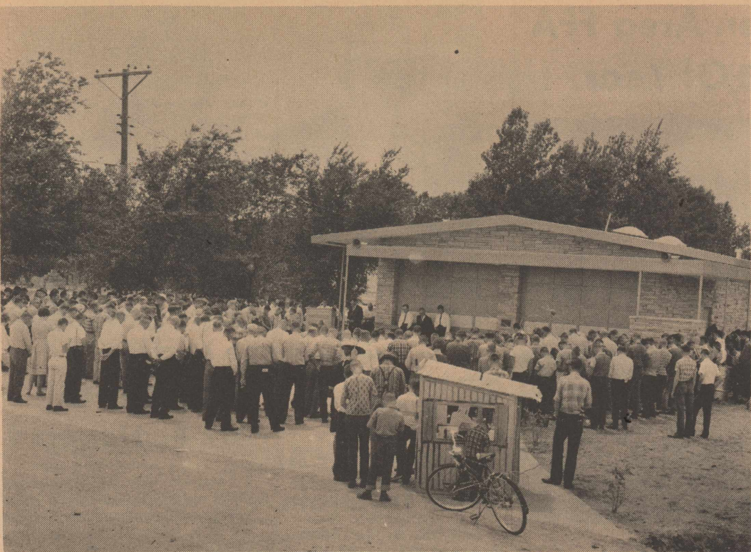
NEW FIRE STATION-Shown above is the new fire station, complete with two new fire trucks, at Boy's Ranch. The dedication was held Saturday. The Olton Fire Department contributed $210 to help purchase the trucks.
