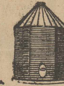
GRAIN STORAGE TANK
