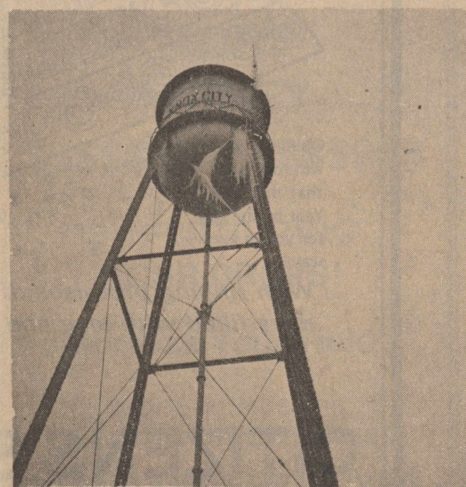
STANDING TALL as a landmark for Knox City, the local water tower also appears to depict the area weather with large ice formations just below the tank Tuesday noon.
