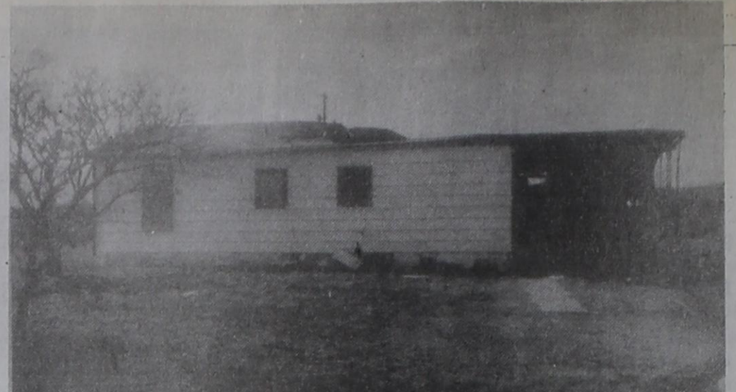
This residence at 4000 FM 2228 about 10 miles southeast of Baird near the Admiral Community was damaged by fire on the morning of December 3. Baird Fire Department contained the fire damage to one room and the attic area.
