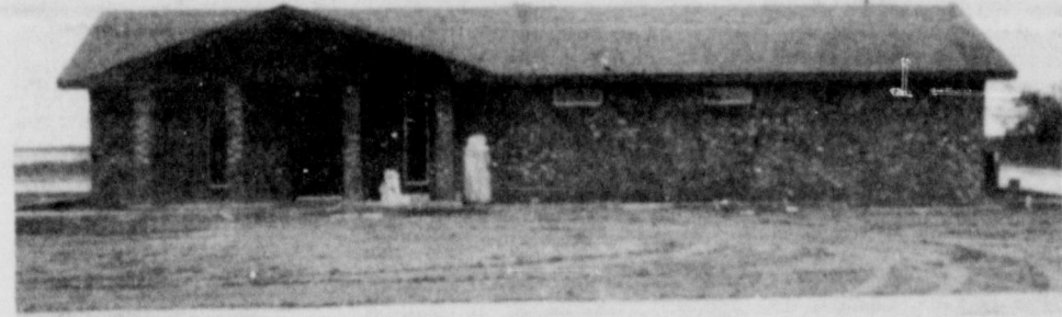
WORKERS ARE FINISHING UP THIS WEEK on the new office building of R.G. Howell, M.D. The attractive building, constructed of antique brick with a dark brown roof, contains 1800 square feet of floor space. Opening date has been set for Monday, April 18.
