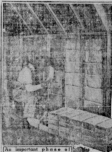
An important phase of America's 1938 building program is home insulation with mineral wool. Because of its efficiency and the ease with which it may be used on both new and old homes, architects and builders recommend complete insulation with mineral wool. At upper left, workman is placing four-inch bats of fire-proof mineral wool between sidewall studs of a new home. At lower right is demonstrated method of filling sidewalls of old houses with mineral wool for year round comfort and economy.
