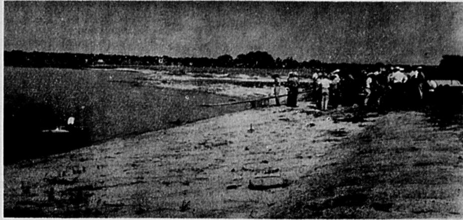
FLOOD PREVENTION SITE — Here is the flood prevention structure which also provides water for irrigation to the Chester E. Woody farm. The site was on recent Callahan County tour to view programs financed in the county by Farmers Home Administration.
