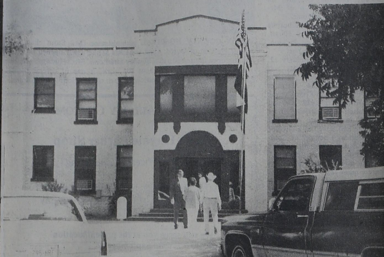
HOSPITAL BOARD TRUSTEE Bill Baker of Knox County (in suit) greets visitors on the walk of the Knox County Hospital at the open house held Sunday afternoon. The hospital re-opened September 1 after being
