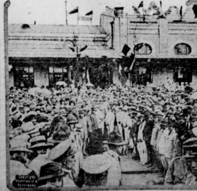
A wonderful ovation was extended to the American troops and other allies upon their arrival in Siberia. Here is shown the railroad station in Harbin profusely decorated upon the occasion of the arrival of the American engineer corps.
