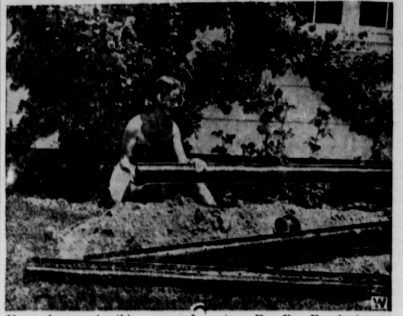
No garden worries this summer for actress Kay Kay Kensington as water flows from a length of lightweight, two-purpose Orangeburg Manufacturing Company perforated bituminized-fibre pipe. It drains a rain and dampens a drought.
