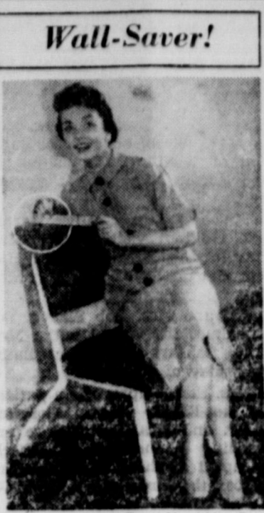
(Courtesy of Royal Metal Mfg. Co.) Here's a new-style chair with a flare for saving walls! The tubular steel chair, introduced recently in Chicago, is designed with flared rear legs which extend beyond its back. Result is a protective space (circle) between chair back and wall, preventing the chair from bumping and marring the wall.
