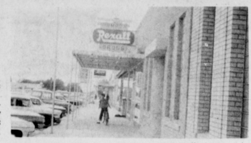
NEW AWNING - Muleshoe's Main Street got another new awning this past week when Damron Drug took on a new look. White's Cashway added a new awning recently, too. (Journal Photo)
