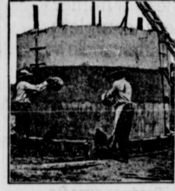
Concrete Silo in Course of Construction.
