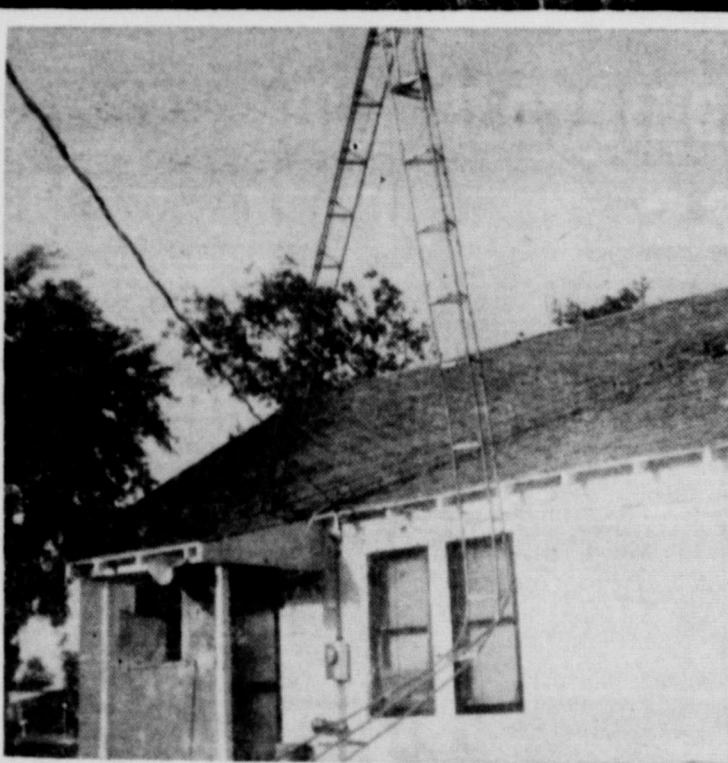
The above picture shows antenna damage caused by a recent windstorm less than 25 miles from Munday. Hundreds more fell across electric lines, in doorways in driveways, etc., causing tremendous damage to property.
