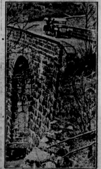
Substantial Stone Culvert.
