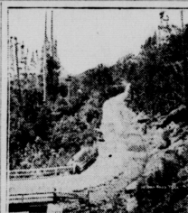
Road Showing Stacks of Stone By the Wayside for Repairs.
