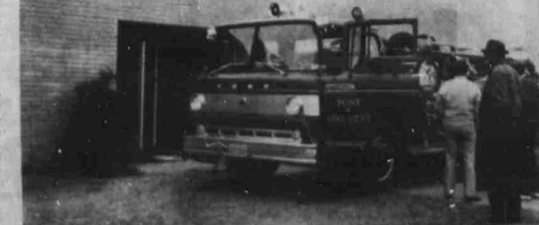
HIGH SCHOOL FIRE — Firemen were called to Post High School at 11:05 a. m. Monday as a precautionary measure because a fire which developed in a heater in the southwest wing of the building produced excessive smoke. "We wanted to be sure it wasn't an electrical fire which could cause expensive damage," Supt. Bill Shiver said. He said damage was confined to the heater itself, and that apparently sawdust sucked into the heater from the nearby industrial arts department had caused all the smoke. — (Staff Photo)
