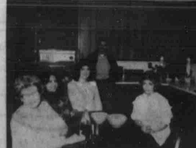
REMODELED KITCHEN — The kitchen has been paneled and new flooring installed. Shown l to r, Sue Shyffles with the Community Action, Susan Valdez, TDHR; Judy Henyan, TDHR; Bob Gibbons and LaVern Howard with TDHR.
