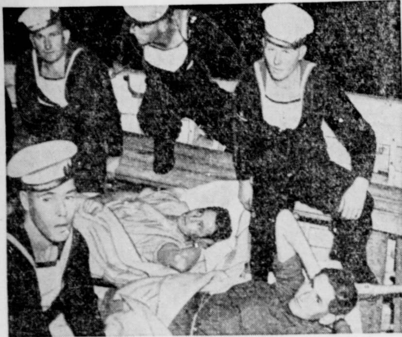
Two Australian seamen, W. D. McBurnie (left) and F. E. Miller, are brought ashore in a lighter at an Australian seaport after being wounded in action in the Solomon Islands. They are survivors of the Australian ship Canberra which was lost in action when American marines and naval units supported by Australian forces made their historic attack on the Japanese-held Solomon Islands.
