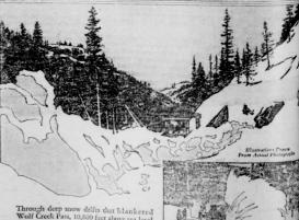
Through deep snow drifts that blanketed Wolf Creek Pass, 10,800 feet above sea level in Colorado's Rockies, a great V-type snow plow doggedly pushed its way. A whirring rotary plow spouted clouds of snow, clearing rotary plow spouted clouds of snow, clearing the roadway. And soon, despite temperatures daily below zero, workers of Liberty Truck & Parts Co., of Denver, had opened the 15-mile road.
