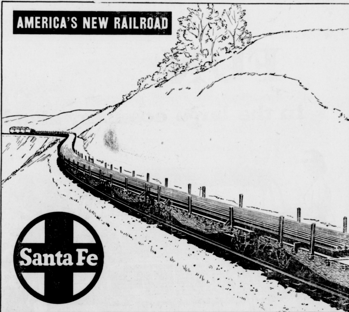
Quarter-mile lengths of welded steel rail curve around a foothill like wire cable.
