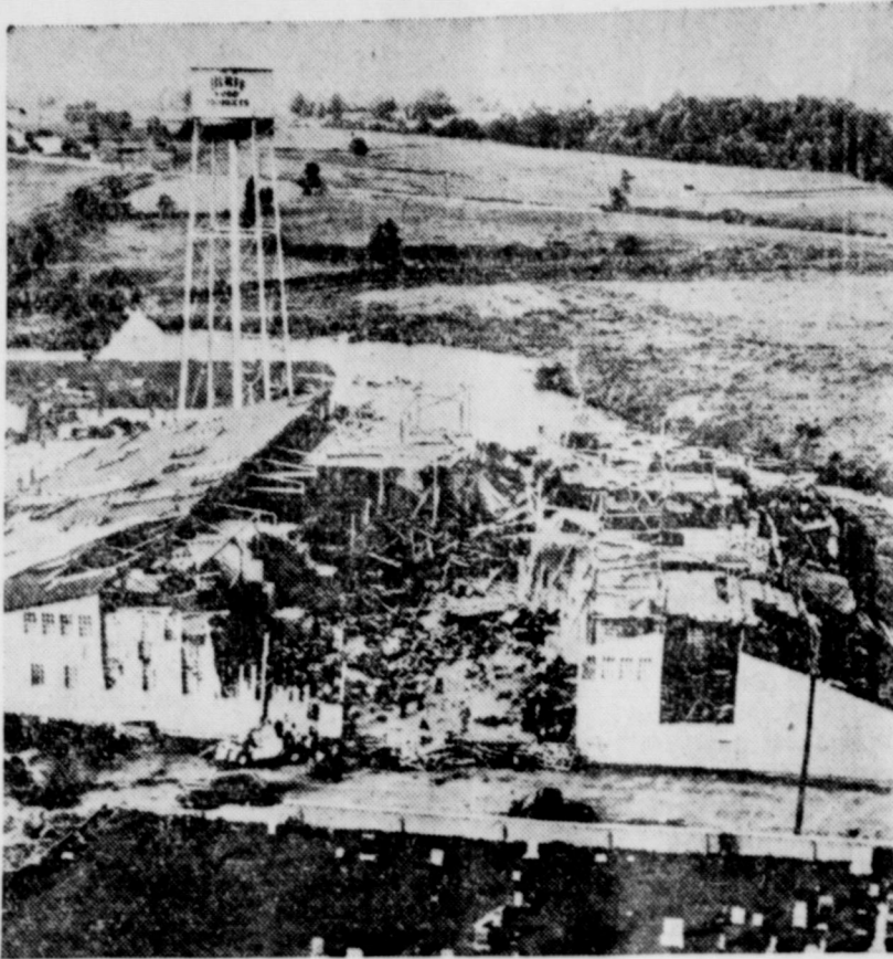
Shown here are the ruins of a cannery factory at Swedesboro, N. J., after a tornado had ripped it to pieces. George Hemple, of Swedesboro, was crushed to death when a 150-foot steel stack at the cannery fell on and smashed the truck in which he was sitting. Eighty others were injured in the cannery. Other sections of Delaware and New Jersey suffered damage from the storm.
