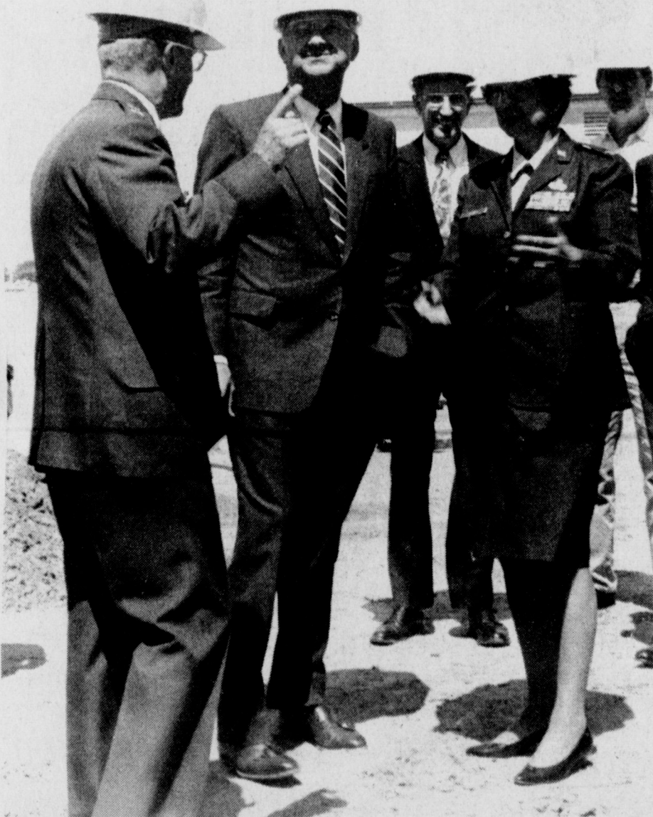
SEN. PHIL GRAMM received an update on construction Tuesday at Sheppard AFB, and a brief tour of one building partially completed. He received input from Gen. Dale Tabor, left, and Col. Karen Konklin. The construction is needed to accommodate numerous new classes to be taught at the base when Chanute and Lowrey bases are closed in the near future. Gramm told the audience the continued enlargement of the air base is assurance it will not be on the closure list for several years to come.
